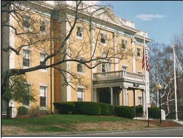
McLean Hospital—Administration Building
